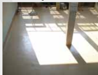
Cooling Tower Basin
