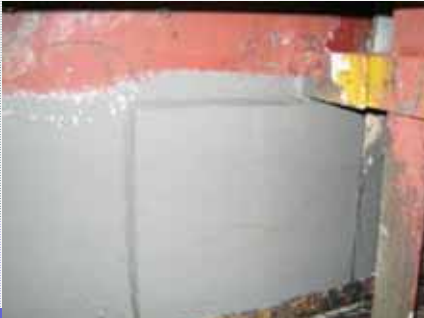
Tank Wall Reinforcement
