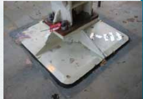
Tank Wall Reinforcement
