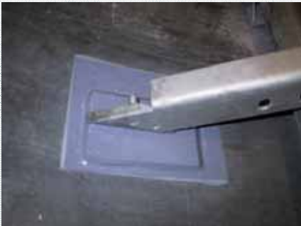
Tank Wall Reinforcement
