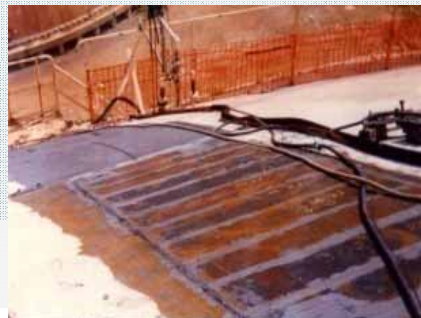
Tank Roof Reinforcement
